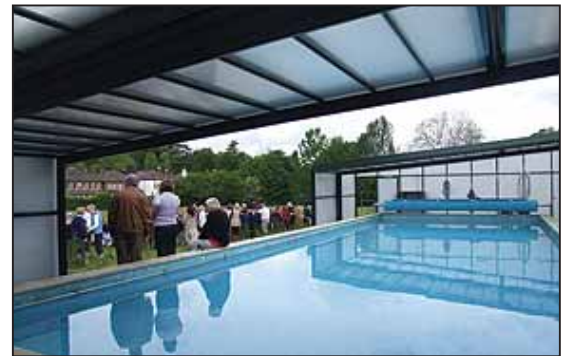
The newly refurbished swimming pool.
