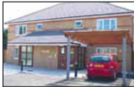
Diana Francis House in Alexander Crescent
