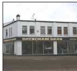
Caterham Cars in Station Avenue has the potential to provide 30 dwellings in the next ten years.
