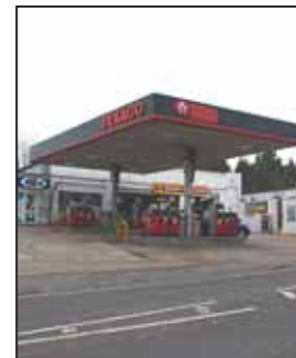
Amongst the commercial sites is the Texaco Garage in the High Street, Caterham-on-the-Hill, allocated eight dwellings.
