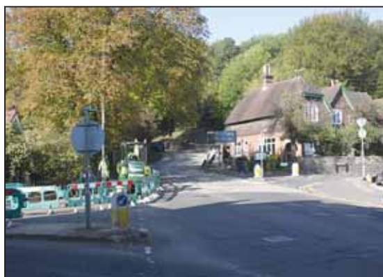
The site of the mini-roundabout under construction in Caterham.
