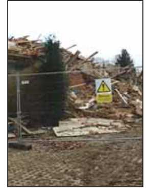
The demolition site in Harestone Valley Road.
