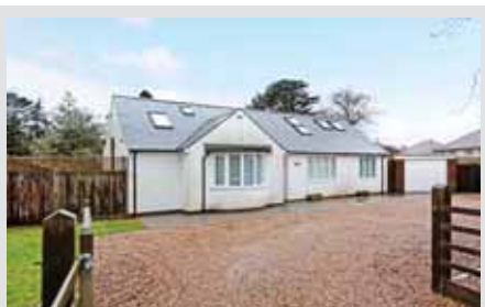
Warlingham OIEO £550,000 Extended bungalow with modern interior. EPC: C Hamptons Caterham & Oxted 01883 759487
