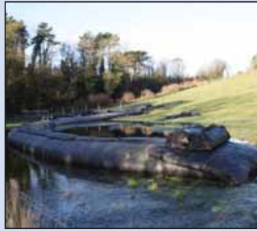
On Friday 21st February the army arrived in Woldingham to create a dam in a field by Woldingham Viaduct. The dam is designed to hold back the flow of the Bourne River to alleviate the flooding in Whyteleafe and Kenley.
