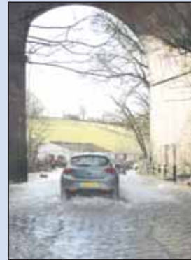
The flood beneath the viaduct in Woldingham.
