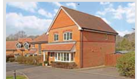
Buxton Place, Caterham OIEO £499,950 A beautifully presented four bedroom detached town house situated in this small and select development built by 'Try Homes' in 2006, offered in excellent condition and with 2 off street parking spaces and lawned rear garden. EPC C Hamptons Caterham & Oxted 01883 759487
